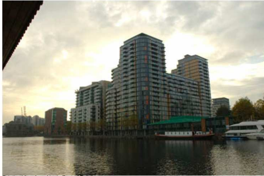
Existing View from North-East of Building
